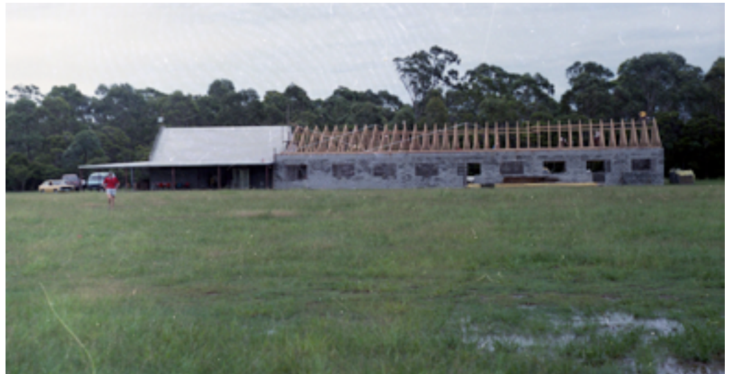
1990: The clubhouse at Willawong under construction.
